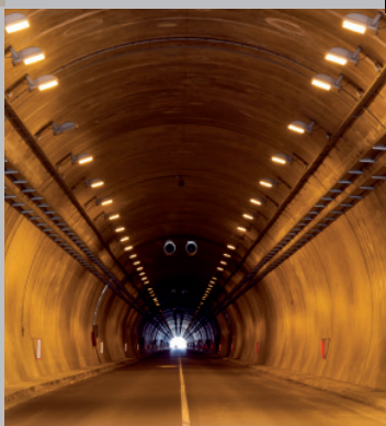
Tunnels and traffic stations
