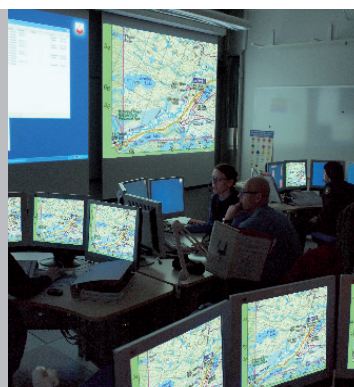
Asset management in control room
